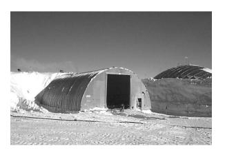
(a) A particular *Wonder Building* has a span of 30 metres and a height of 10 metres. Find the radius of the arc.
